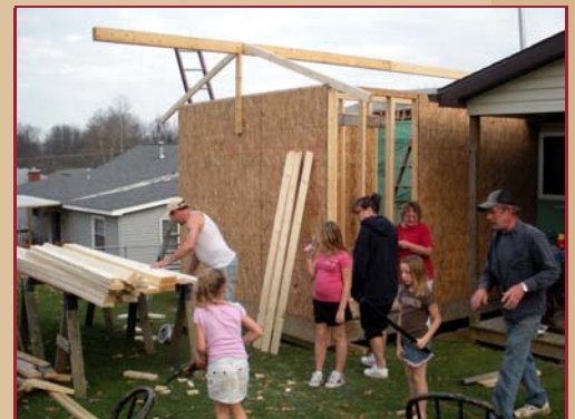
The family works together to build a new room.
